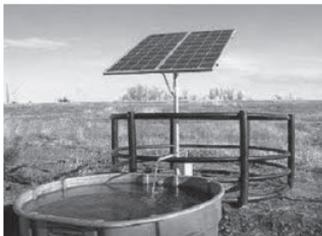
Figure 12: Solar Water Pump
