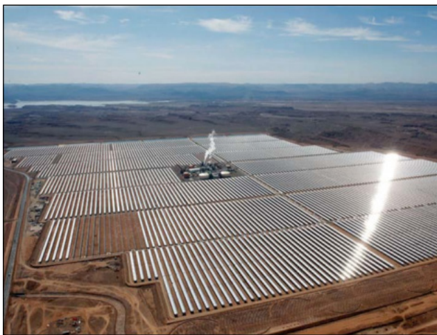
Fig. 12: Overview of the largest solar power plant (Morocco)
